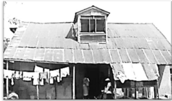
Plate 4: Dormer window in Apete compound, No.50 Ìta-Olóókan Street, Osogbo which earned the building "the house with spectacular decoration" (Photo: F.M. Abéjidé, 2019).
